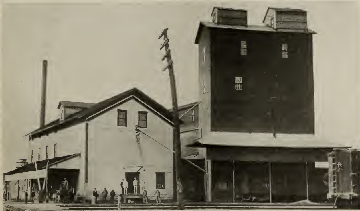
ELEVATOR AND MILL OF THE E. E. DELP COMPANY, BOURBON, IND.
